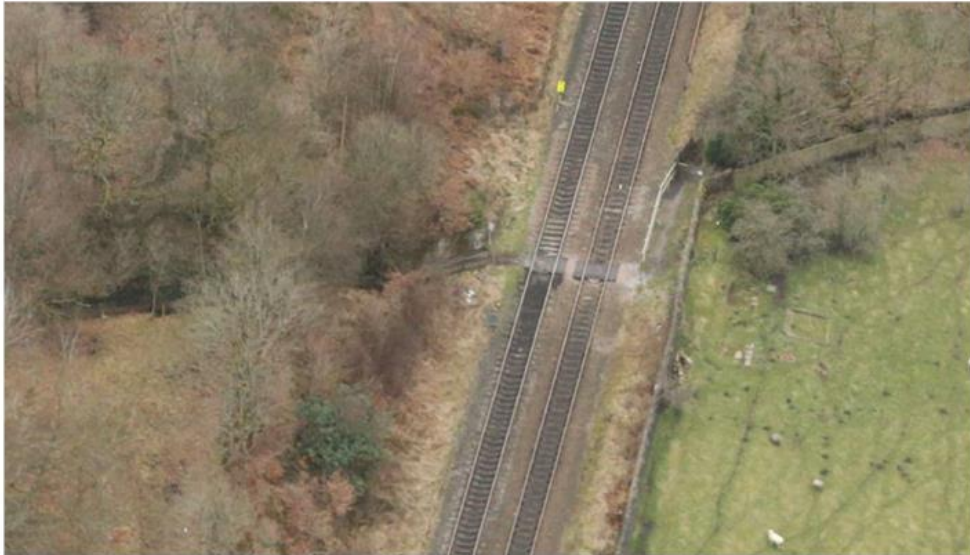
Ariel view of Moorgate Halt LC
